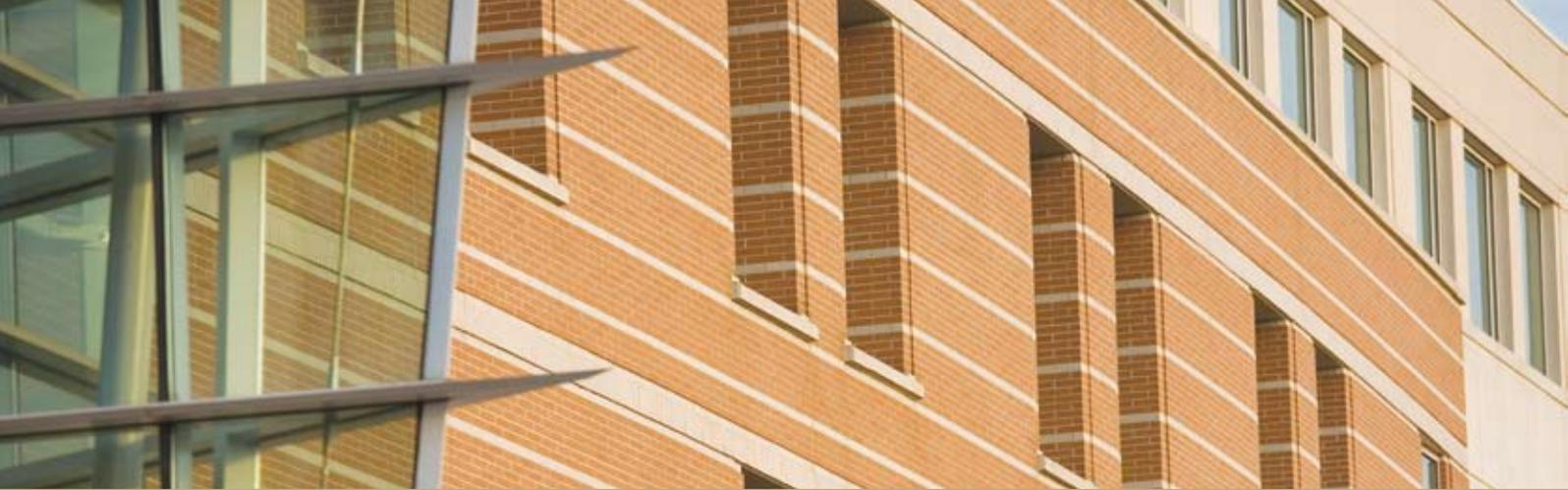
**BLENDING** Belden takes the extra manufacturing step of factory-blending its brick. That way we can control and randomize minor color variations and assure color consistency in the finished structure. Our blending procedure means brick can be laid up just as it comes off the package without concern for concentrated color variances.
