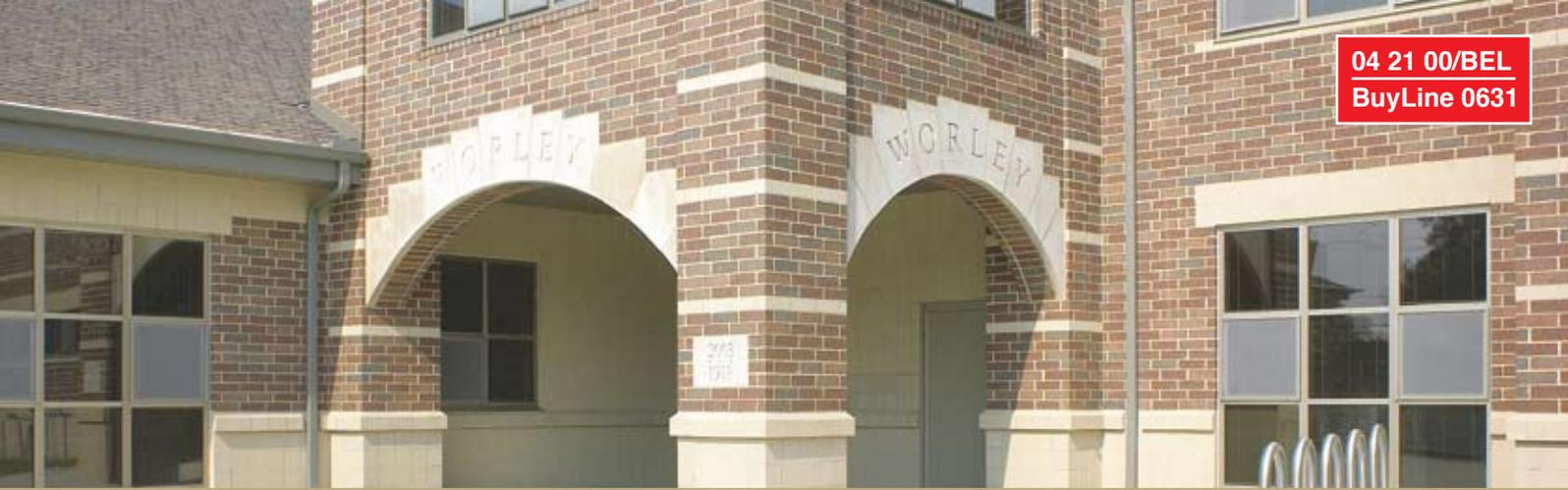
**TEXTURES & SIZES** Belden Brick is offered in textures that range from the sand mold finish of colonial times to rugged randomly textured styles... vertically grooved styles or silky finishes. Each texture can make its own distinctive contribution to the visual impact you seek. Belden Brick is regularly manufactured in sixteen different sizes. Representative dimensions and related information are provided on pages 10 and 11.
